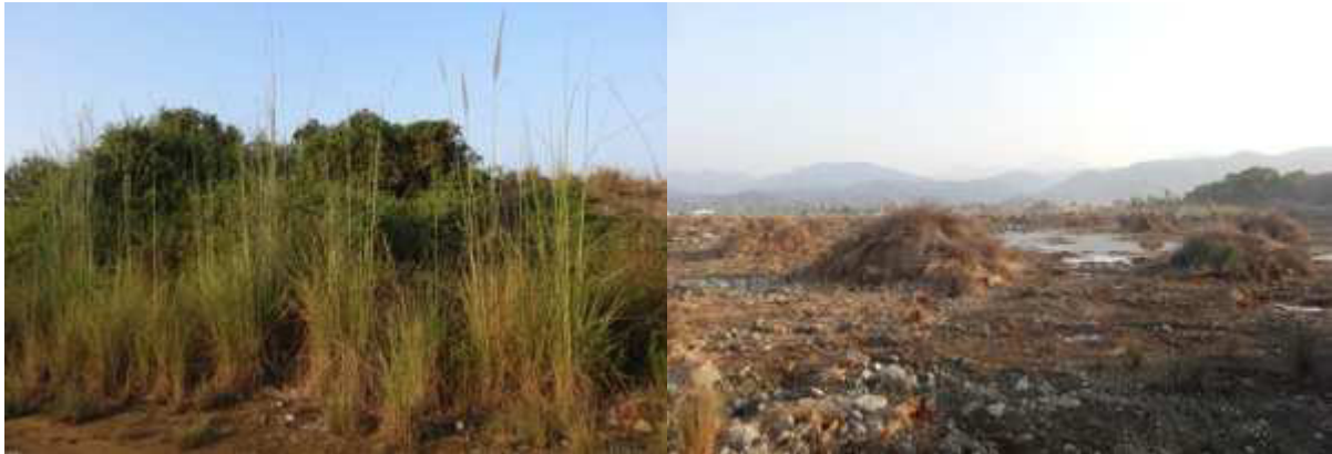
Fig. 60: Wetland next to the construction site before and after being bulldozed (Photo: M. Herzog)
