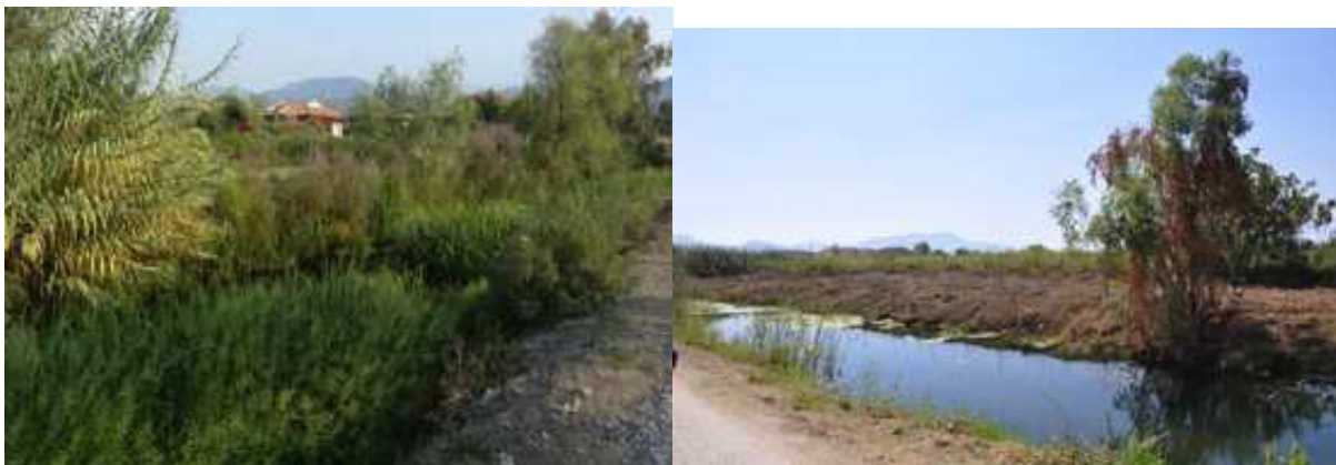
Fig. 61: Reed belt next to the construction site before and after bulldozing (Photo: M. Herzog, M. Stachowitsch)
