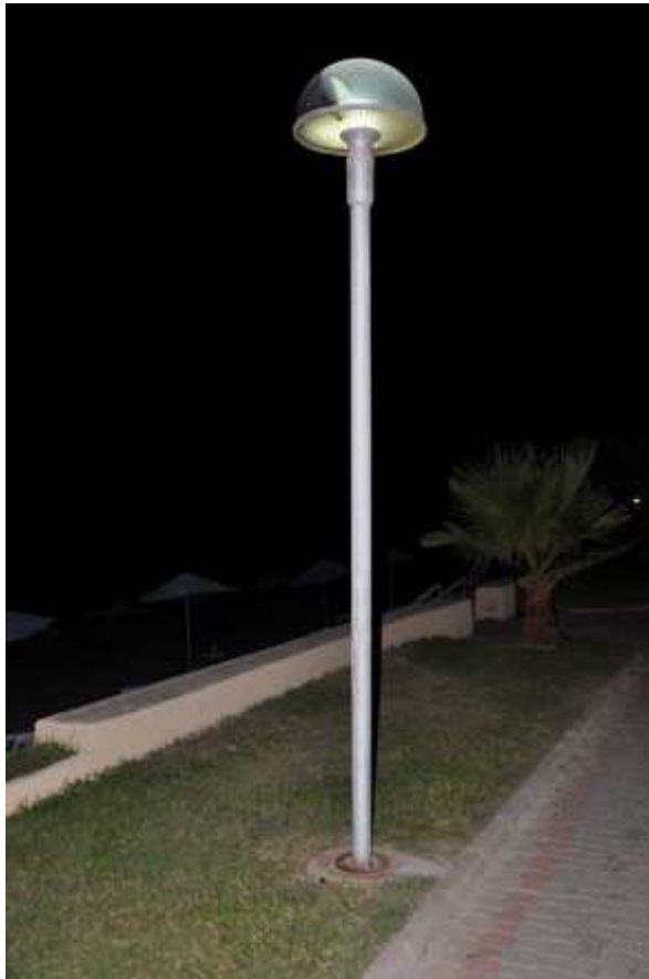
Figure 4: One of the 24 street lamps along the promenade with a technical modification to (partially) block the light from the beach. (Photo: M. Stachowitsch)
