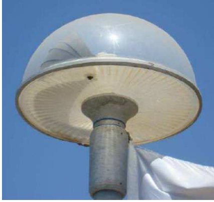
Fig. 4: Lantern on the beach of Çalış with beach-facing part partially shielded (Photo: B. Böswart) Abb. 4: Laterne mit Abschirmung am Strand von Çalış
